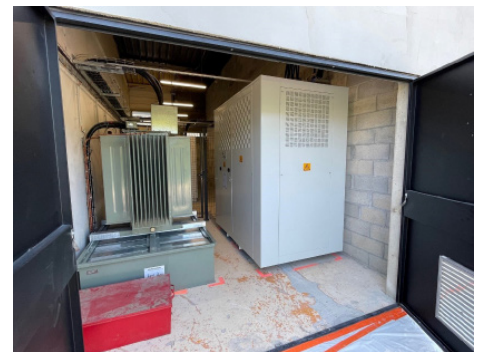
Low voltage switchboard with our HV/LV transformers in the background
