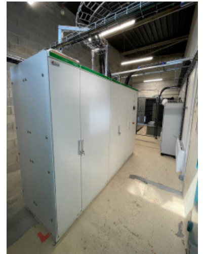
Low voltage switchboard with our HV/LV transformers in the background
